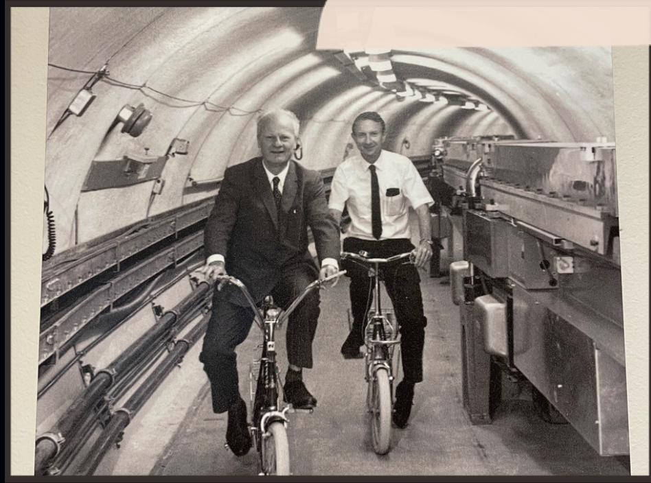
Image From Manhattan Project National Historical Park Los Alamos
